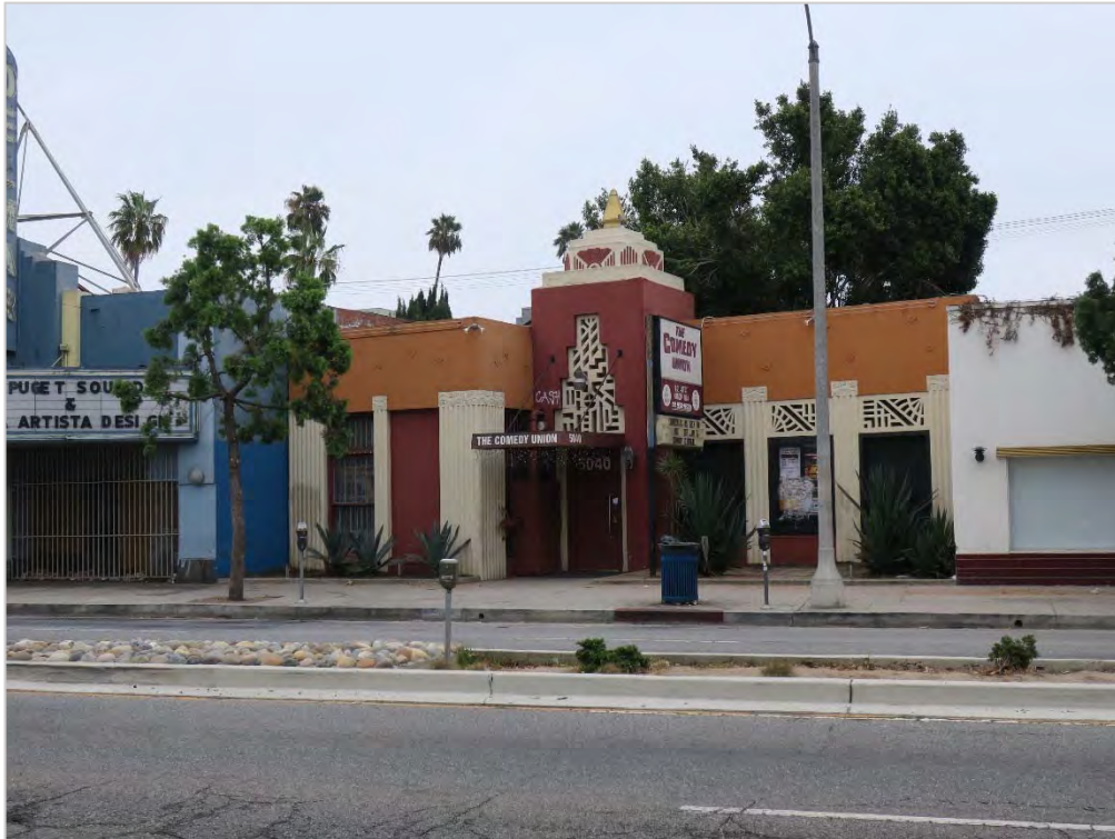
Primary (north) façade, view south (ARG, 2017).
