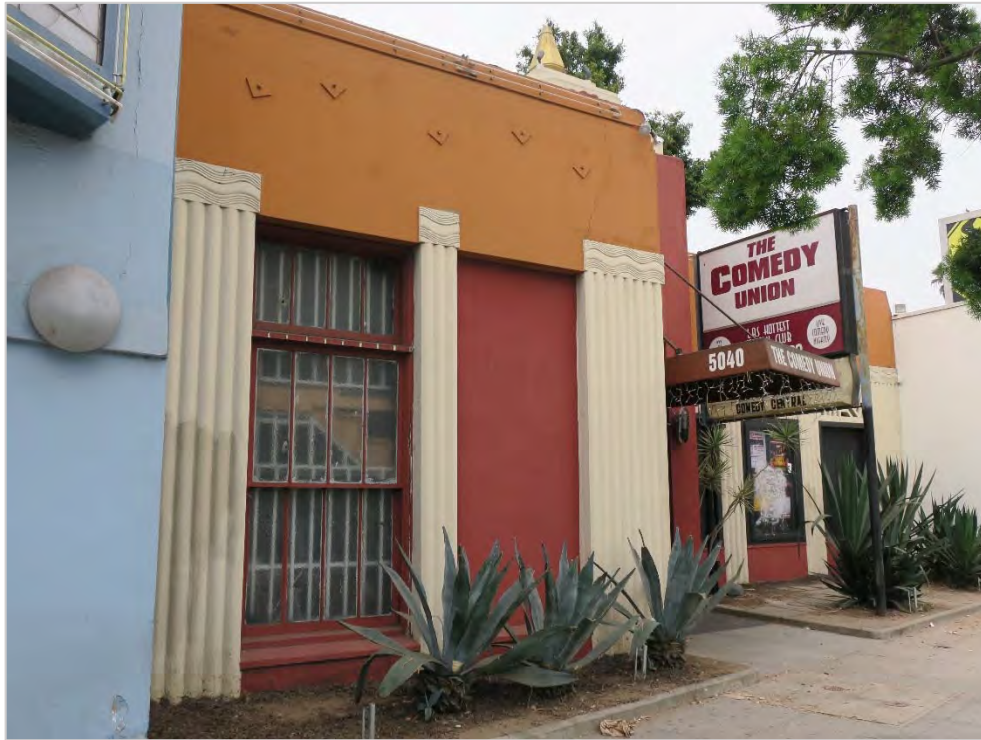
Detail of steel double-hung window on primary (north) façade (ARG, 2017).
