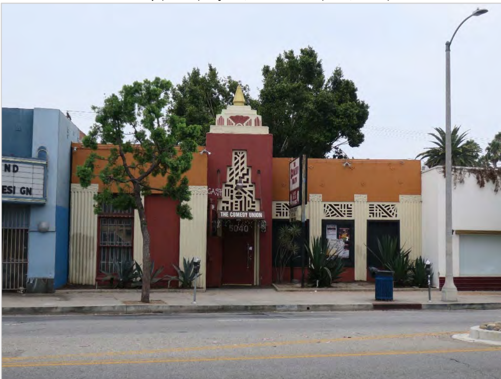
Primary (north) façade, view south (ARG, 2017).
